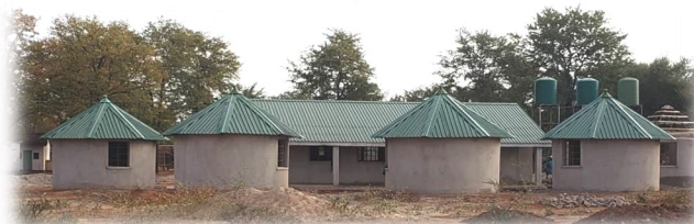
Waiting Mother’s Village under construction
